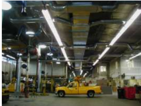
City of Los Angeles Building Modifications & Methane Gas Detection
